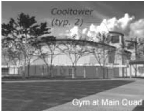
at the base of the tower that opens into the space to be conditioned. Operable windows or louvers high within the conditioned space work together with the tower to complete the system. To start, the roll-up door and windows/louvers are opened and the water pump turned on. As air passes through the
